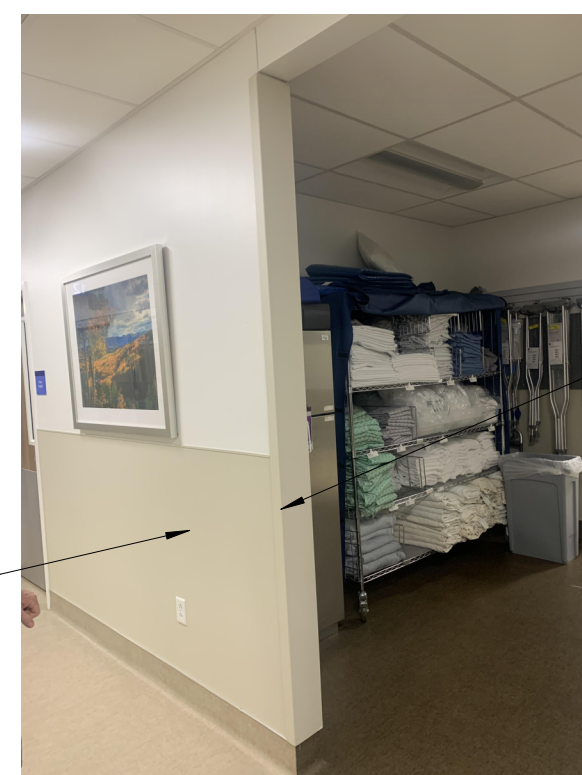
WALL PROTECTION / GYP BD TO BE REMOVED
